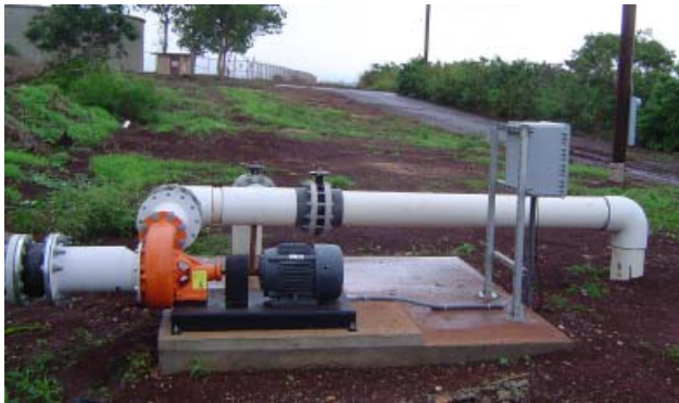
Newly installed pump-back station at Reservoir 225 in the Waiahole Irrigation System.
